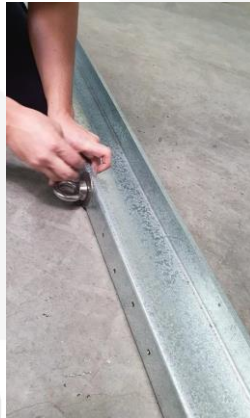
Step-5: Install the Eyebolt through 700D Washer, Purlin then RafterLink plate.
