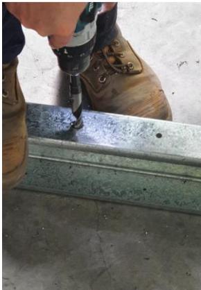
Step-4: Use 16mm drill bit to drill hole at eyebolt location.
