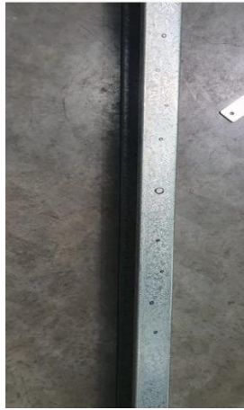
Step-2: After marking all the holes, remove the RafterLink plate.
