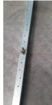
Step-6: Place Spring Washer and Nut to fix the Eyebolt and tighten the nut. Note: Before tightening the locking hex nut turn the eyebolt to line up with the purlin.
