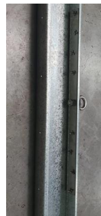
Step-9: Check installed correctly and tighten nut. Threads need to have a minimum of six full 360° turns into the ultimate thread.
