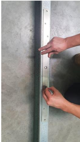
Step-1: Position the RafterLink plate at installation location and mark all the holes.
