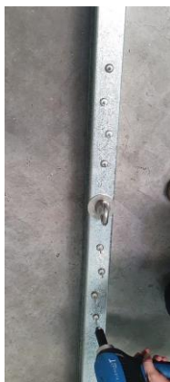
Step-7: Position all rivets into drilled holes.
